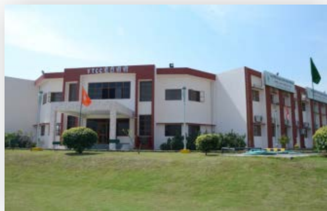
1 st phase VTCC Building
