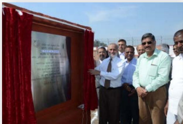
Secretary DARE and DG ICAR laying Foundation Stone for BSL-3 facility of VTCC
