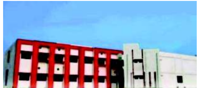
VTCC laboratory under construction
