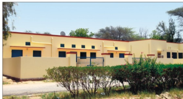
Renovation of the staff quarters
